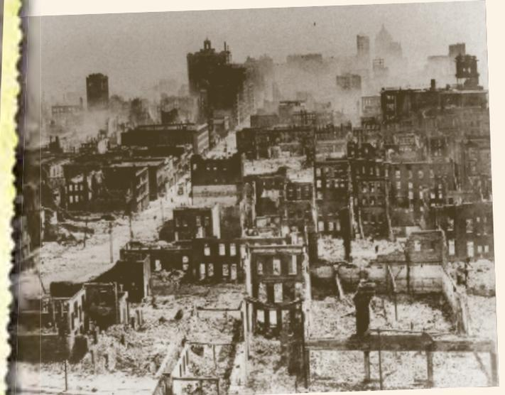
The shifting of the earth during the quake caused underground pipes to rupture. Some of those pipes carried natural gas, a highly flammable fuel. The leaking gas caused fires. Other broken pipes were water mains—and when the mains broke, that meant that firefighters had no water to use to fight the fires. Unchecked, the fires spread quickly.
